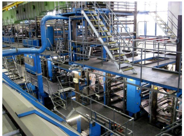
A Goss HT70 Press installed at the Ellerslie print centre
